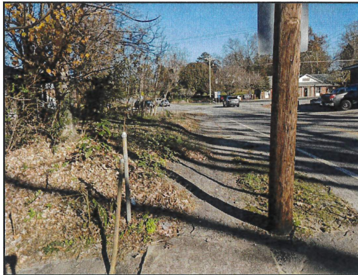
Continuation of sidewalk on Main Avenue West – note the gap between the crosswalk pictured above and the continuation of sidewalk below. The resulting terrain of the gap is hazardous for pedestrians.
